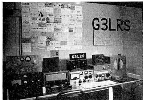
The Leicester Radio Society's shack. The equipment at G3LRS is an Elizabethan transmitter, a 50 watt modulator, an Edystone 680X, a 10 watt NFD tx and a 10 watt Top Band tx.
